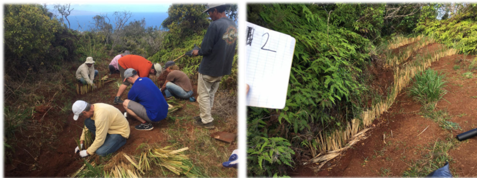
Figure 2-29. West Maui erosion control in watershed using vetiver grass to catch sedimentation. Planting vetiver rows (left); finished vetiver rows (right). Source: West Maui Ridge to Reef
