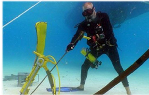
Figure 2-43. A diver installs a mooring buoy on the seafloor. Source: NOAA
