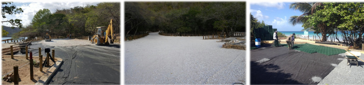
Figure 2-40. Examples of low-impact development practices and permeable parking areas that allow for filtration of rain/runoff. Source: Protectores de Cuencas
