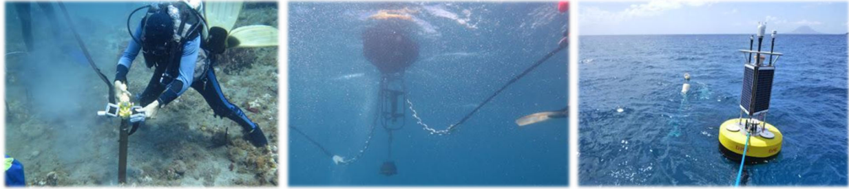
Figure 2-9. CREWS buoy installation. Left: The core barrel drill; Center: Buoy before attachment underneath the water; Right: buoy above water. Source: NOAA Atlantic Oceanographic and Meteorological Laboratory
