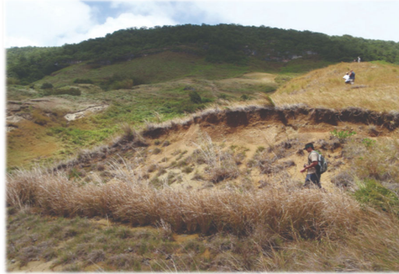
Figure 2-28. Volunteers plant vetiver grass to stabilize soil in the Talakahaya watershed in Rota, Commonwealth of the Northern Mariana Islands. Source: NOAA
