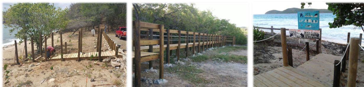
Figure 2-41. Examples of elevated boardwalks and delimitation of sensitive vegetation areas while allowing public access to beaches. Source: Protectores de Cuencas
