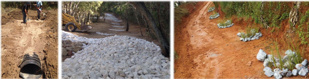
Figure 2-33. Dirt road stabilization in Puerto Rico. Source: Protectores de Cuencas
